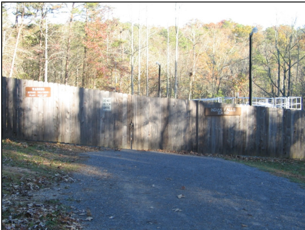
sewage treatment plant in DeSoto State Park
