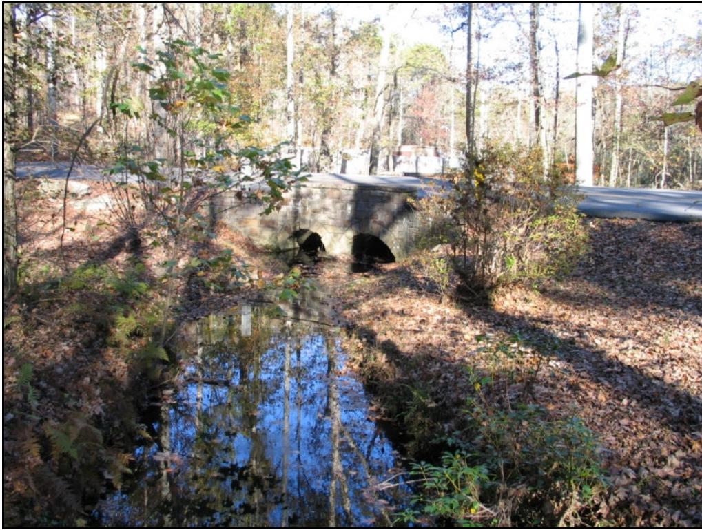
DeSoto Parkway crossing unnamed tributary
