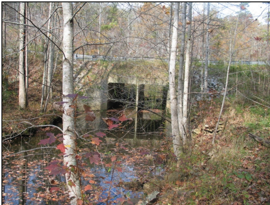
State Route 176 crossing Wolf Creek
