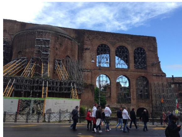
(f) Structural Bracing of Historic Building
